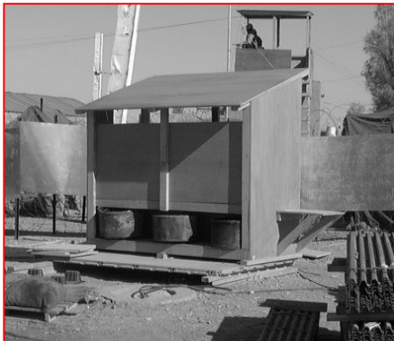
Figure 2. Burn-Barrel Latrine
